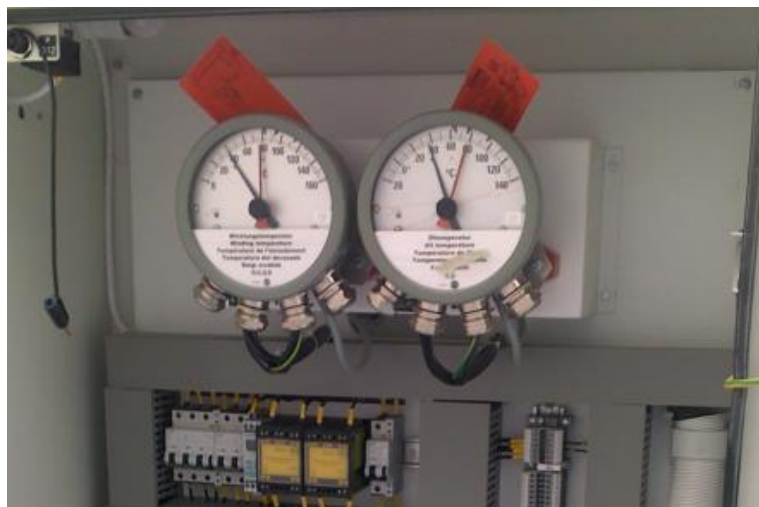
Figure 2. Gas density monitoring indicator
