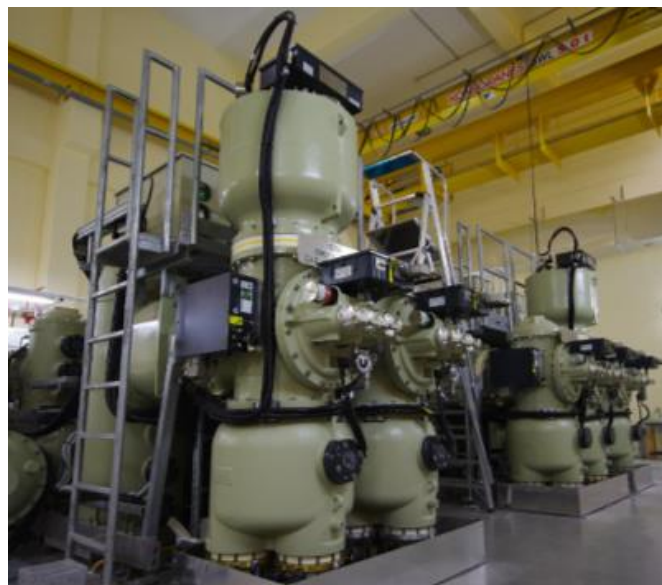
Figure 1. Ladders and platforms in GIS
